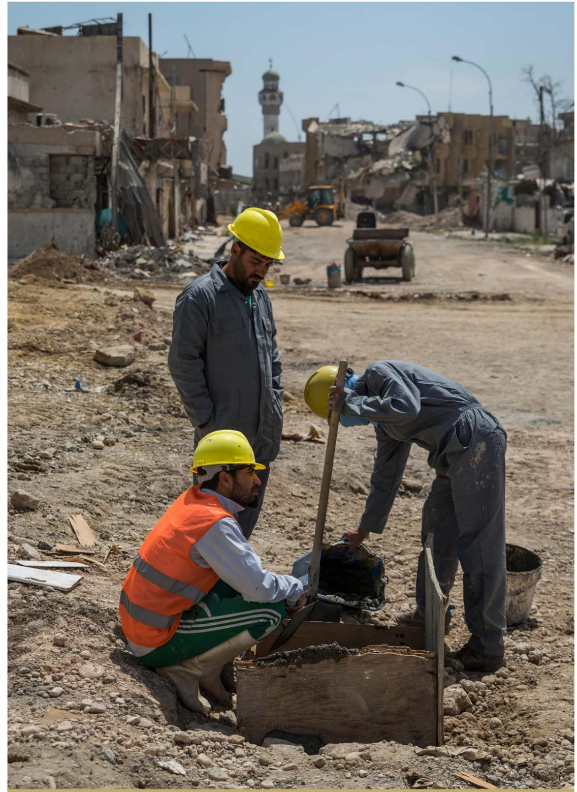
WORK IS UNDERWAY TO REPAIR THE SHIFAA SEWERAGE SYSTEM IN THE WEST MOSUL HOSPITAL COMPLEX.
